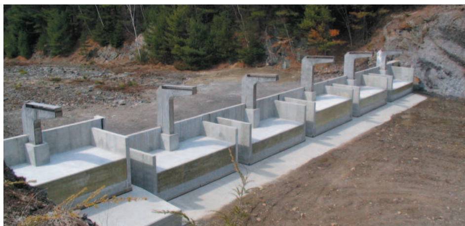
View looking downstream
