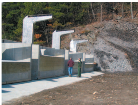
Close view of Otterbrook Fusegates
