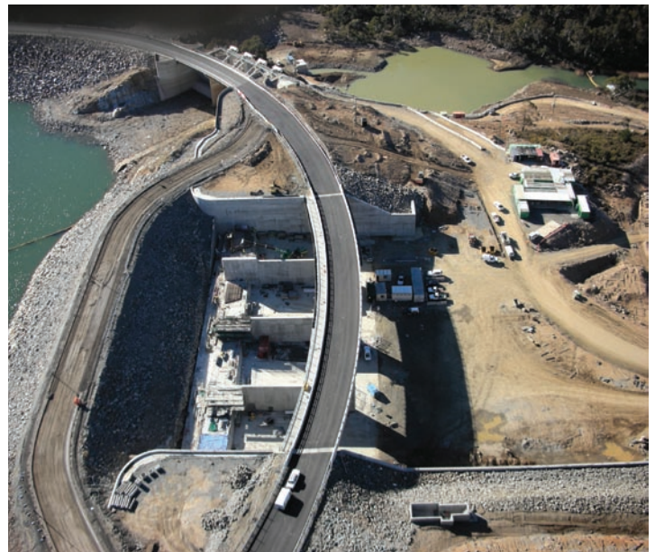
Aerial View of the works
