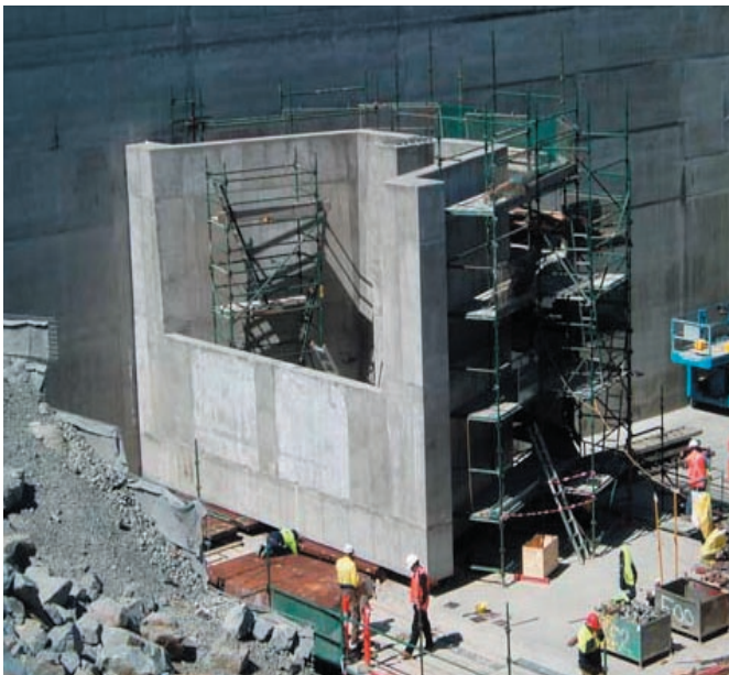
View looking downstream
