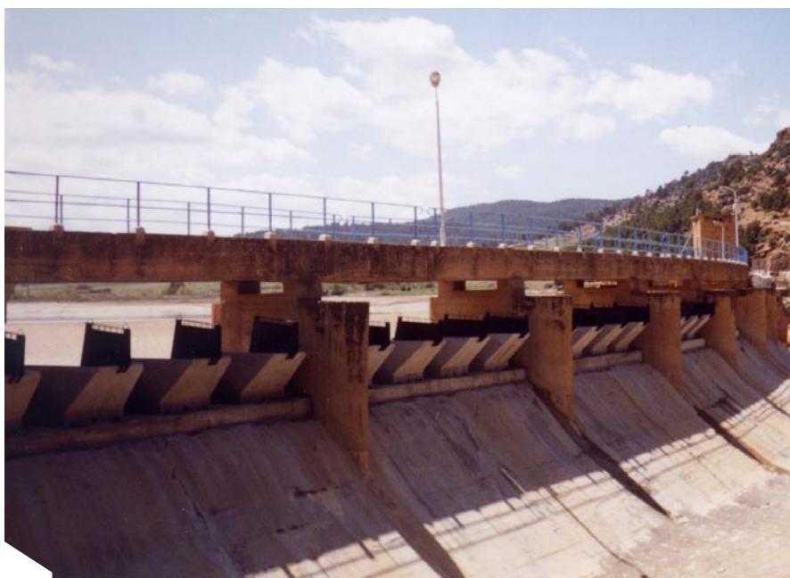
Foum el Gueiss is a rockfill dam, 23 m in height, built in the 1930s. It features a free sill with a curvature centred on the upstream side and a walkway atop the supporting piers. The dam is located upstream Kais, 80 km east of Batna.
