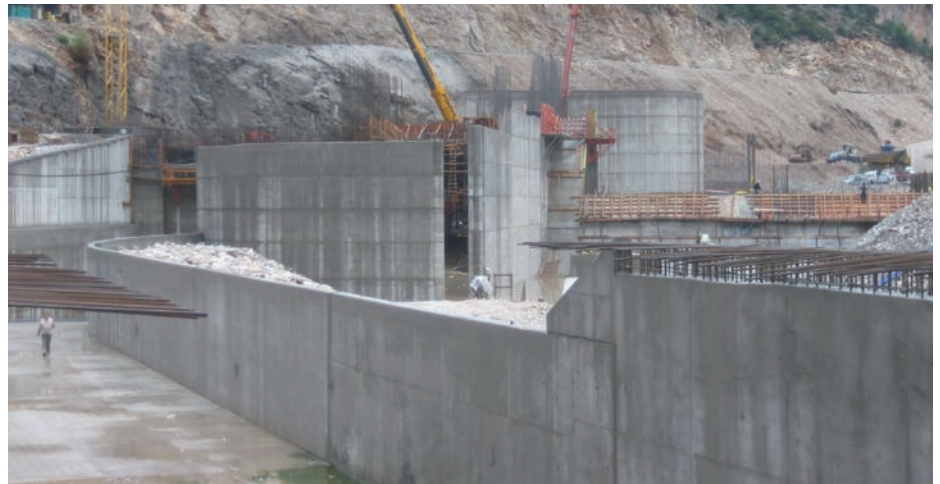
Dafnozouara dam under construction.
