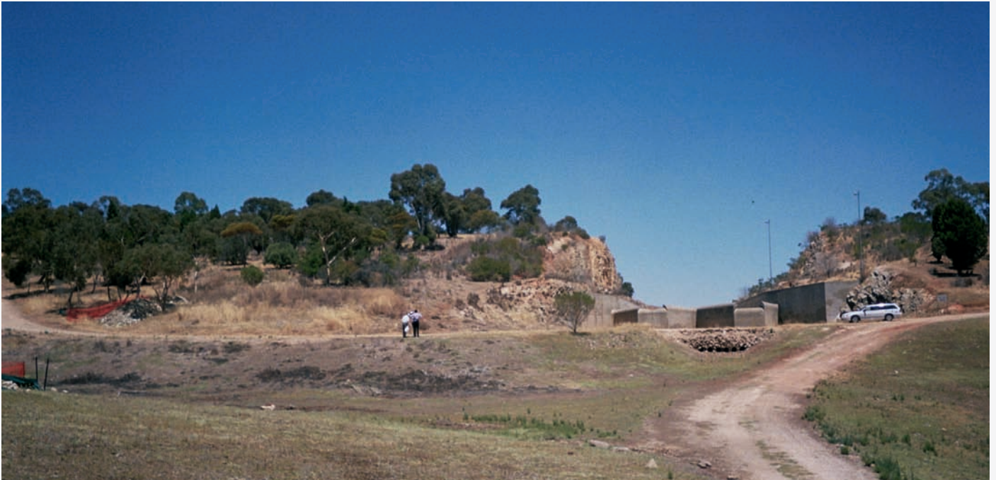
Little Para's existing service spillway and to its left position for excavation of new Fusegated auxiliary spillway.
