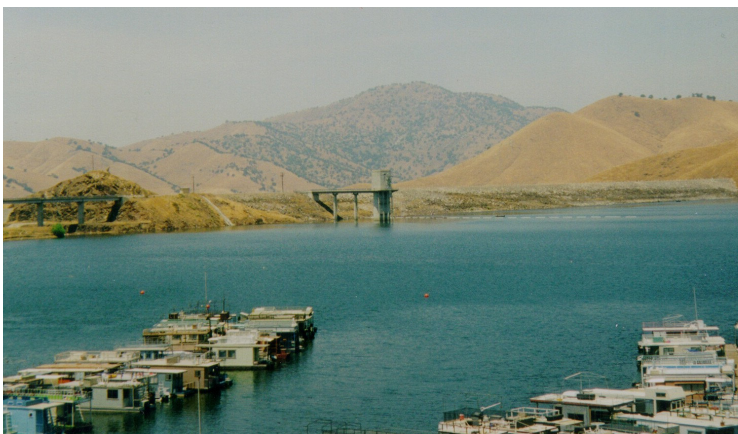
Upstream View of the Dam and Spillway
