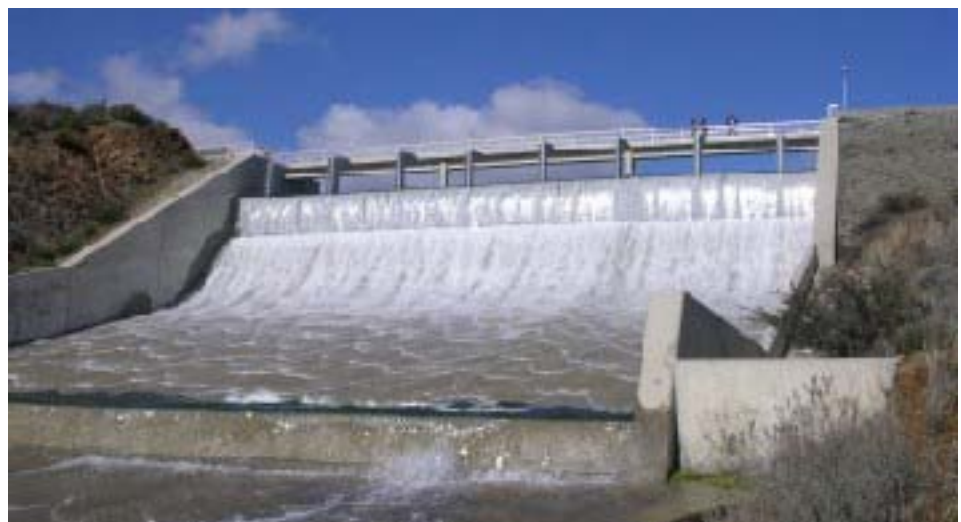
DHYPOTAMOS DAM OVERSPILLING
