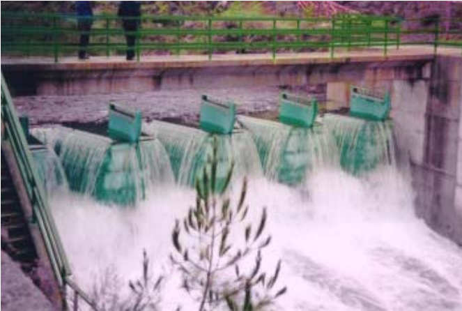
XYLIATOS DAM OVERSPILLING
