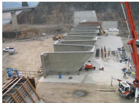
Figure 10. View of Fusegates under construction
