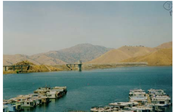
Fig. 2 Upstream view of Terminus Dam
