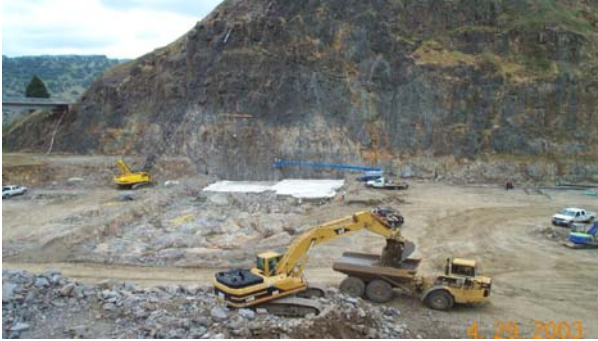
Figure 5. Excavation for Fusegate Foundation
