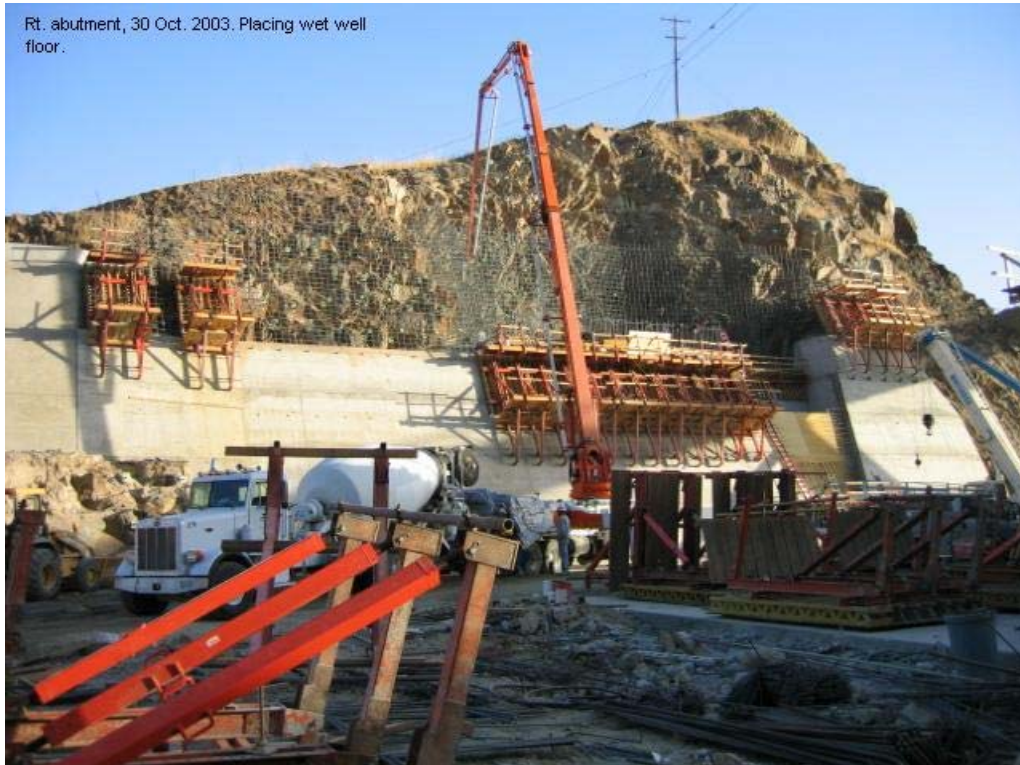
Figure 11. Concreting works for the Intake Tower at the right abutment
