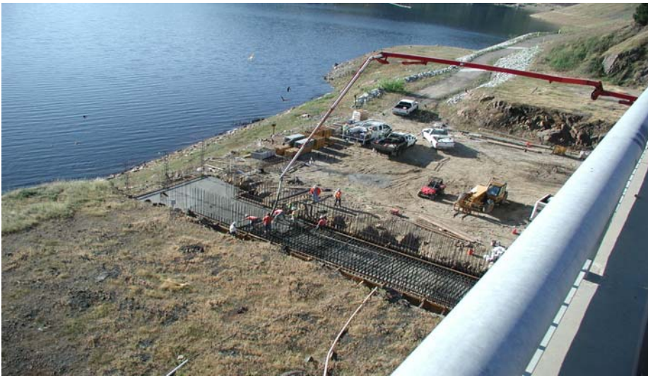
Figure 7. Construction of Intake Structure and the conduit
