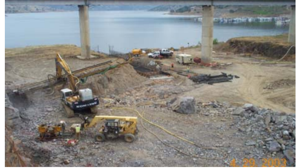
Figure 6. Removal of Benches at the spillway
