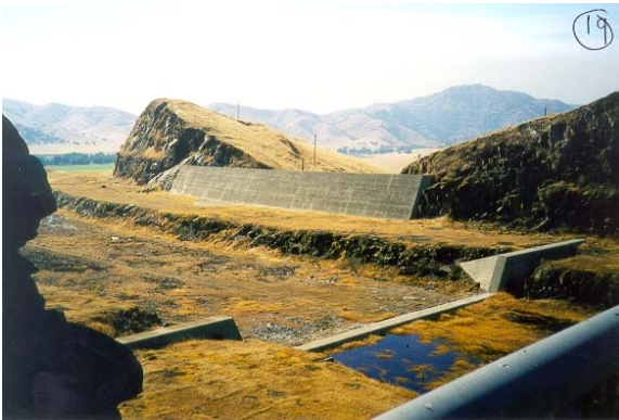
Fig.1 Existing Spillway weir and channel
