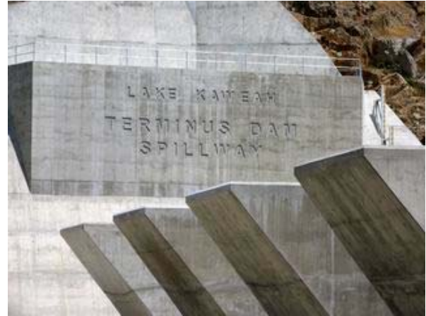
Figure 13: View of Fusegates from the left abutment
