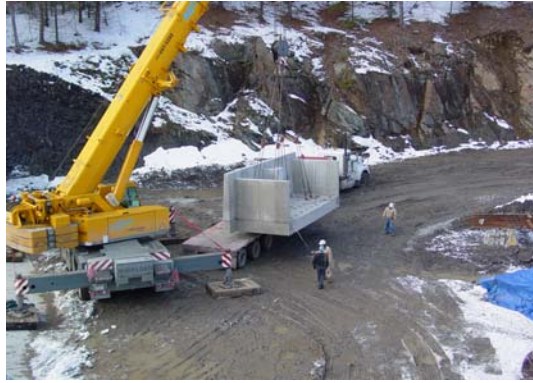
Fig. 6 Pre-cast Fusegates transported to the site
