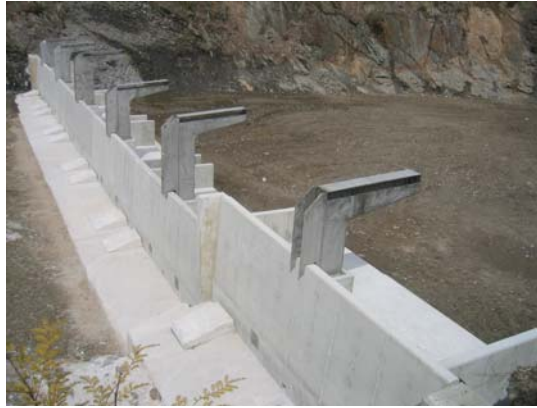
Fig. 10 Upstream view of Fusegates
