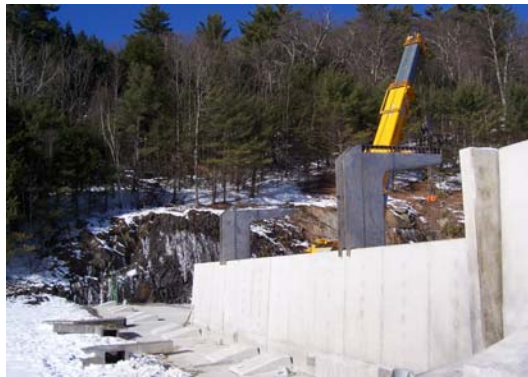
Fig. 7 Downstream view of Fusegates and lugs
