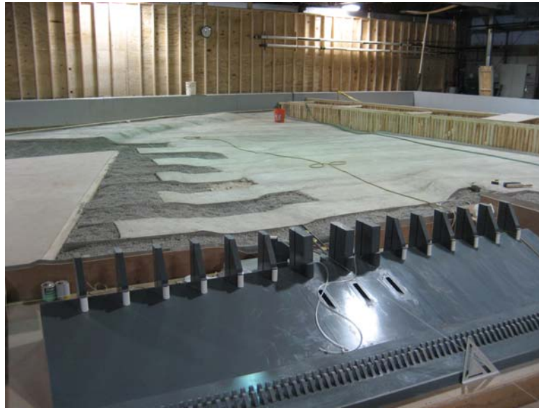
Fig. 19 Canton Dam physical model under construction at Alden
