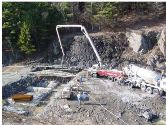
Fig. 5 Construction of the new sill
