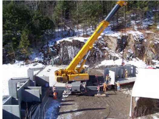
Fig. 8 Upstream view during installation
