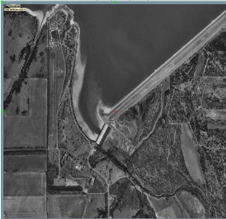
Fig. 11 Satellite view of the Canton dam service spillway
