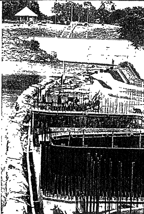
Figure 5 Construction des hausses pendant la période des crues Construction of fusegates during flood periods
